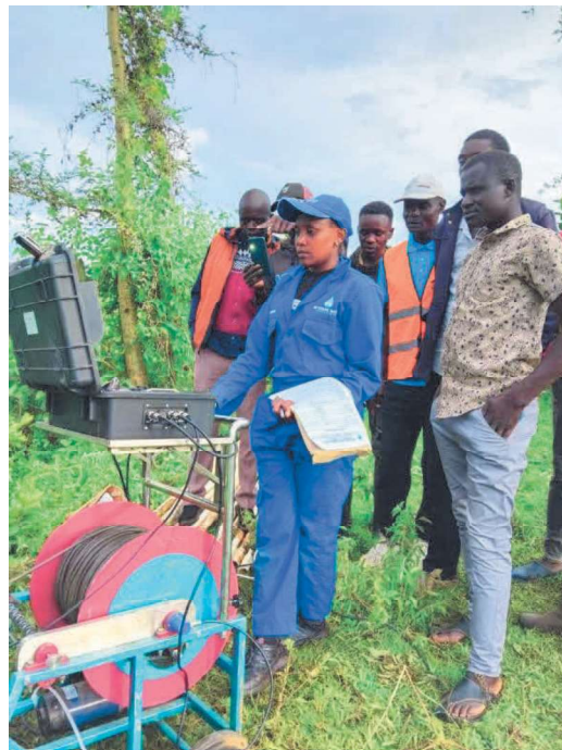
Figure 11: Camera Inspection Ongoing
