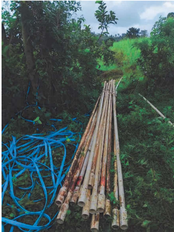
Figure 5: Lifted Pipes and Cable
